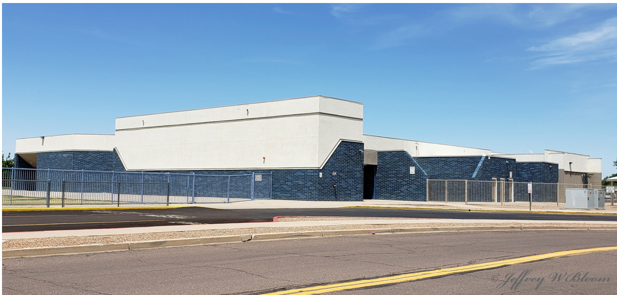
Windowless elementary school in 2024.
